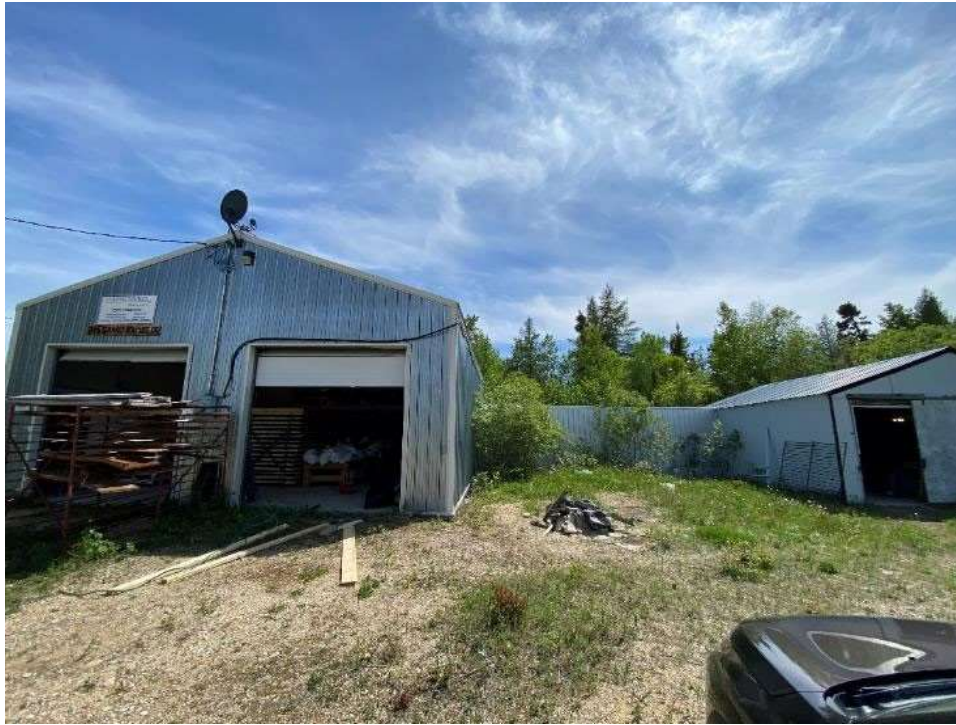
Figure 12-3: Core processing facility
